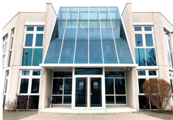
Our new location at Walheimer Str. 2 in Bietigheim-Bissingen
